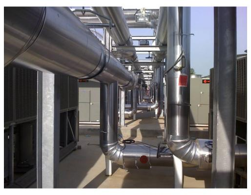
This customer had several data centers that needed insulation for its chilled water supply & return and hot water supply & return, for a total of 34,000 linear ft. The scope of insulation work for the three data centers combined was \$3.92 million.
